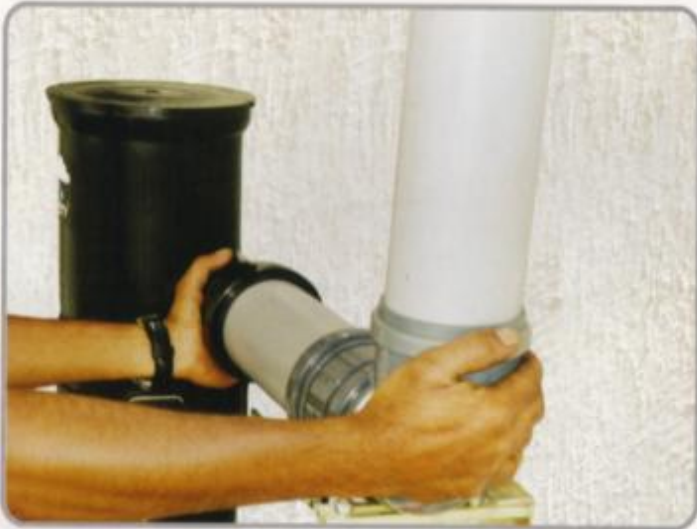
5. Connect the down take Pipe to the inlet of the Filter.
