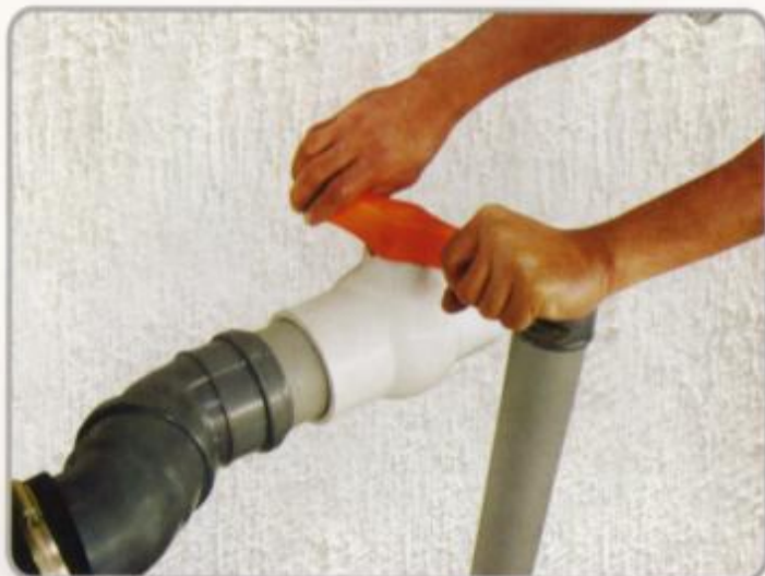
9. When the rainy season ends, close the control valve, so as to make the sudden summer season rainwater go to the drain.
