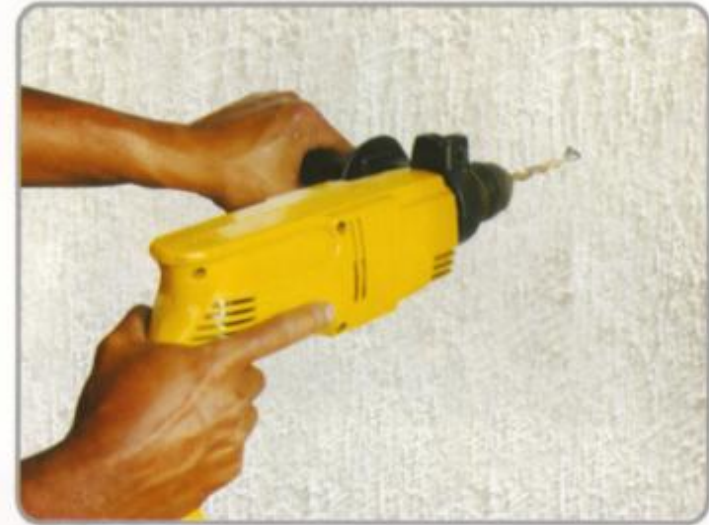
5. Drill the holes to the wall as per the marking.
