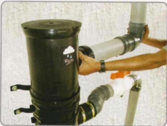
6. Use push type of Elbow with suitable coupler and required length of Pipes.
