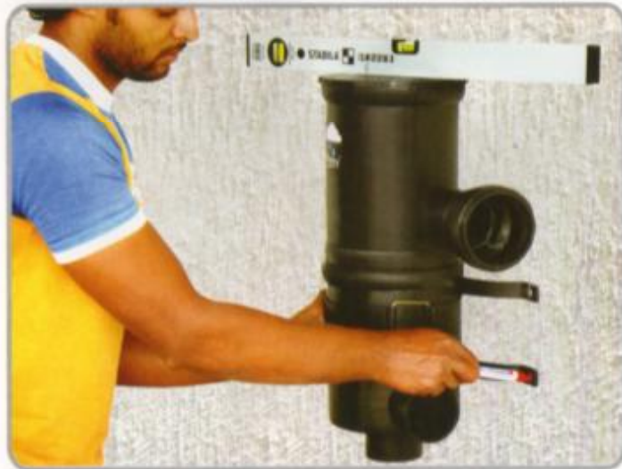
4. Place the filter against the wall to spirit level as shown in the figure and mark the point to fix the wall bracket
