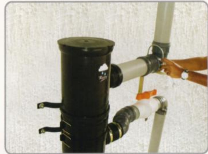
7. Fix "L" angular Clamps with "U" clamps and anchor bolts with adjustable "C"- Channel.
